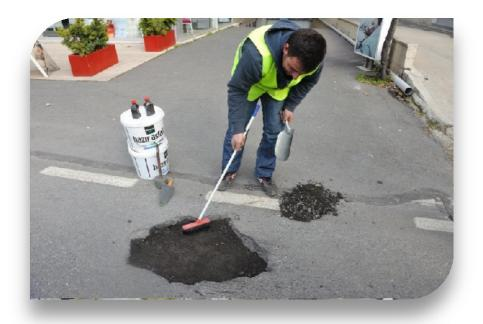
Clean out all debris and loose material from the base. Remove any standing water and wait until the surface is dry.
