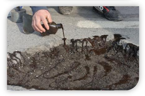
Emulsion, which is supplied with cold mix asphalt, is applied to the bottom and sides of the pit with the help of a brush or roller and let stand for about 5 minutes.
