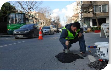
Compact asphalt mixture using hand rammer, compactor or roller. Compaction can also be done by passing over it with vehicles.
