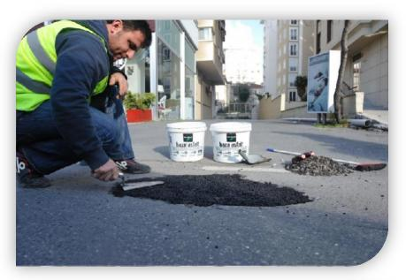
Pour the material into the pit and spread out with a shovel to cover the defected area, slightly mounding. After this process, asphalt is smoothed by hitting it with a shovel or similar tool.
